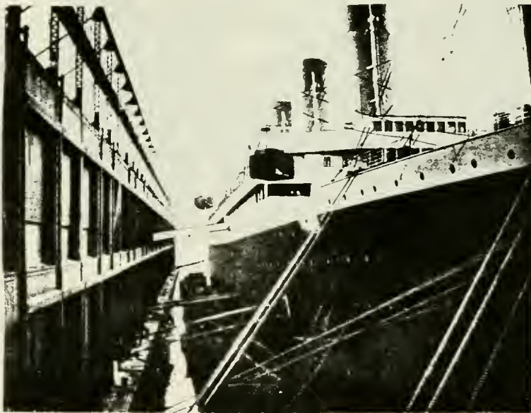
FIGURE 4.4 Burtoning system in use. From Cunningham, Cargo Handling at Ports , 1924, facing page 74.
